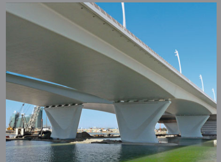
Al Garhoud Bridge, Dubai (AE)
